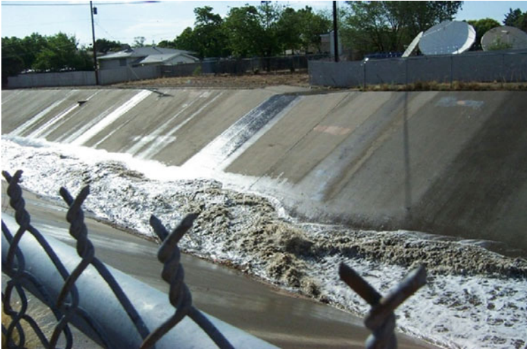
Fig. 2.4. Simple hydraulic jump occurring in a flood mitigation channel in Albuquerque, New Mexico, USA (Photo courtesy of Albuquerque Metropolitan Arroyo Flood Control Authority).
