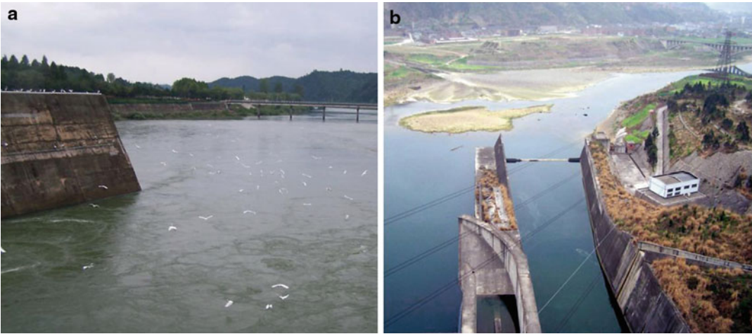
Fig. 3.16. (a) Birds are searching for dead fish at the outlets of a hydropower plant at which fish are killed when they swim through the turbine; (b) The Baozhushi Dam on the Bailong River has cut off the flow and greatly affects the stream ecology in the lower reaches.
